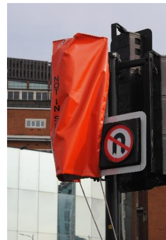
correct bagging of signal heads
